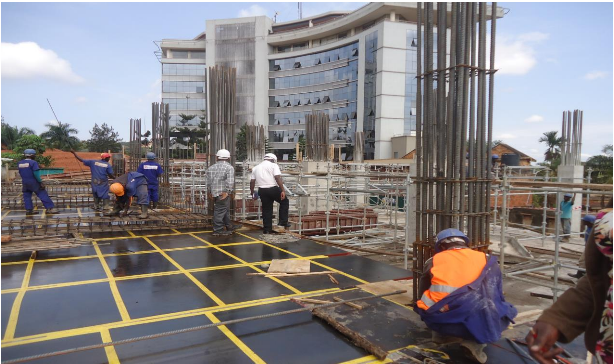
Figure II showing ground floor slab preparation for casting
