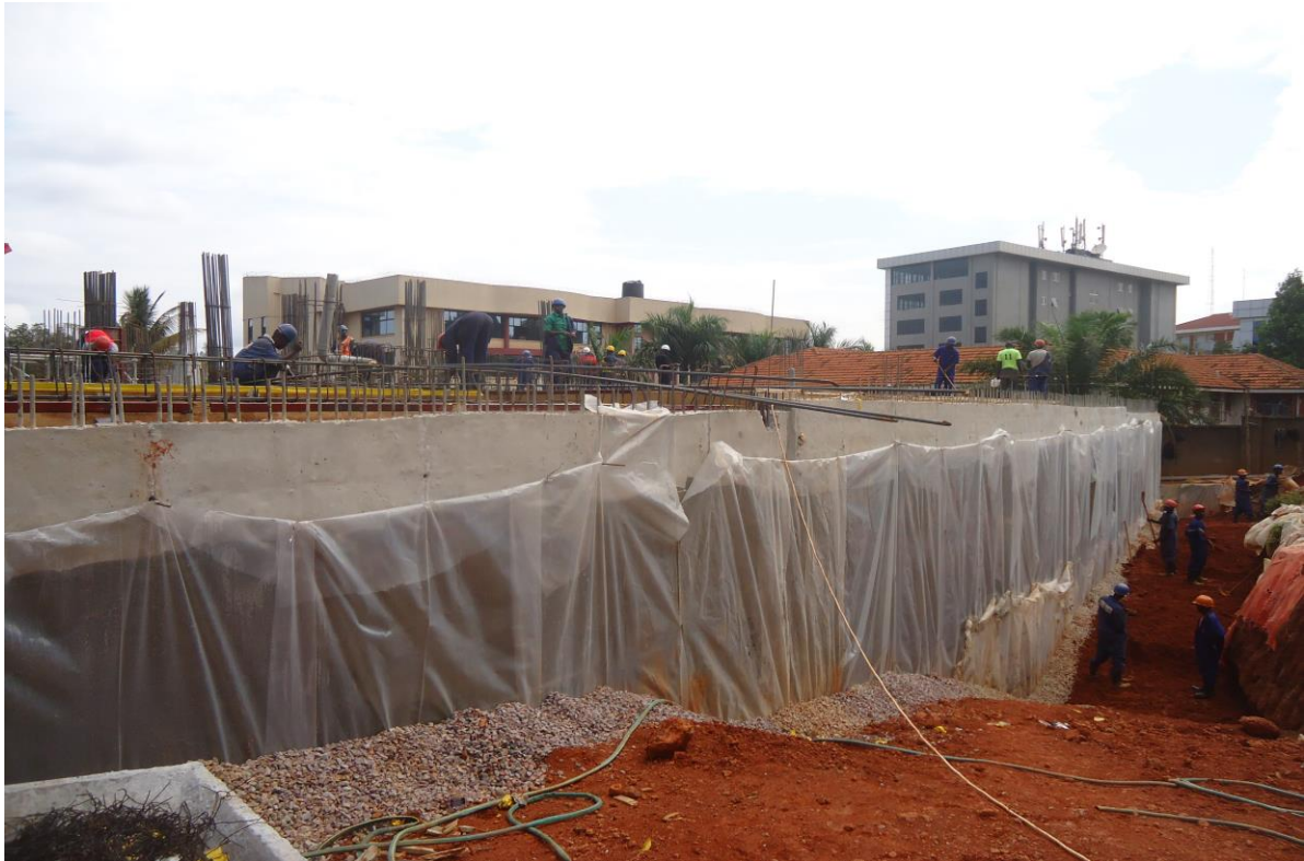
Figure III showing back filling around the retaining wall
