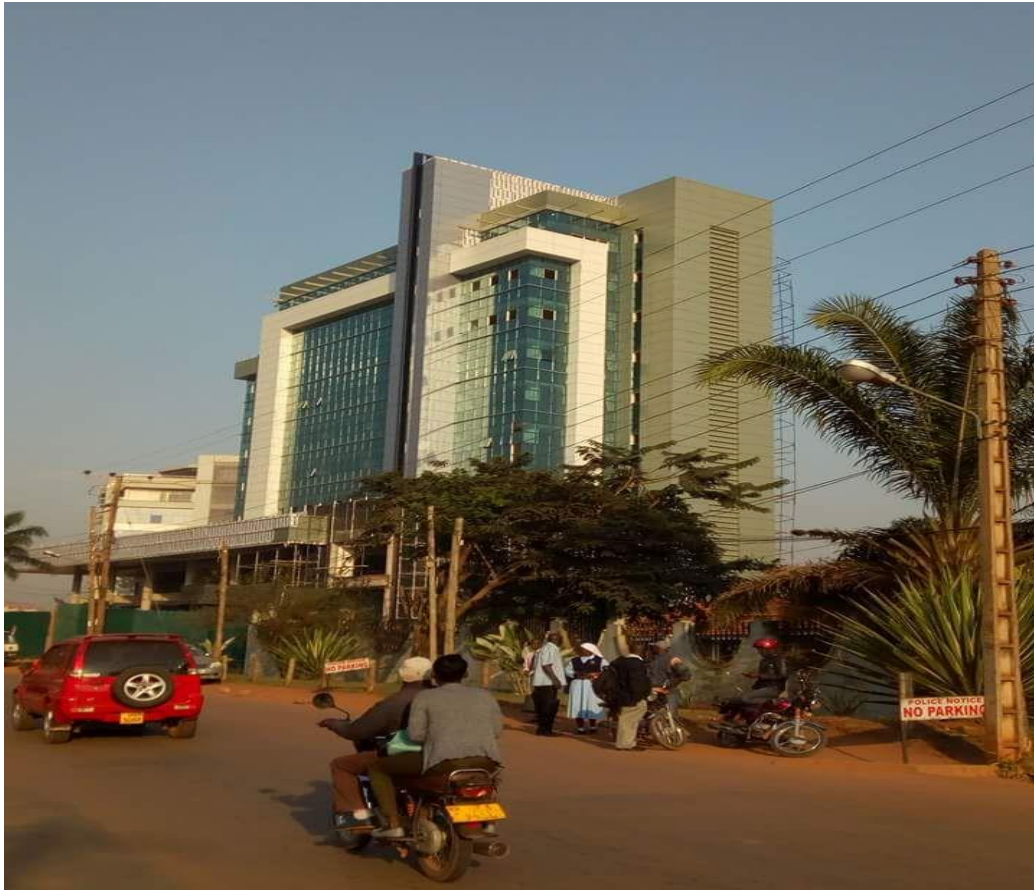
Figure V showing finished sama plaza
