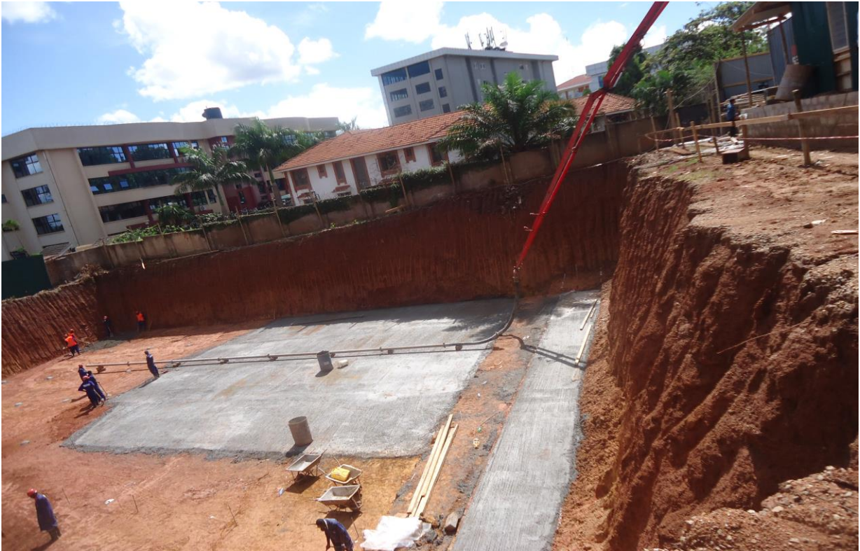
Figure I showing concrete blinding to receive the raft foundation
