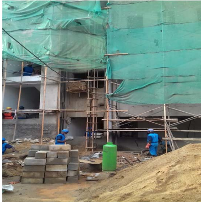
Figure 11: Material and Hoist Machine
