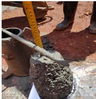
Figure 13: Slump test for concrete
