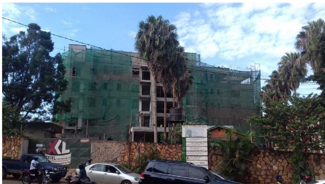
Figure 5: Site Progress in elevation
